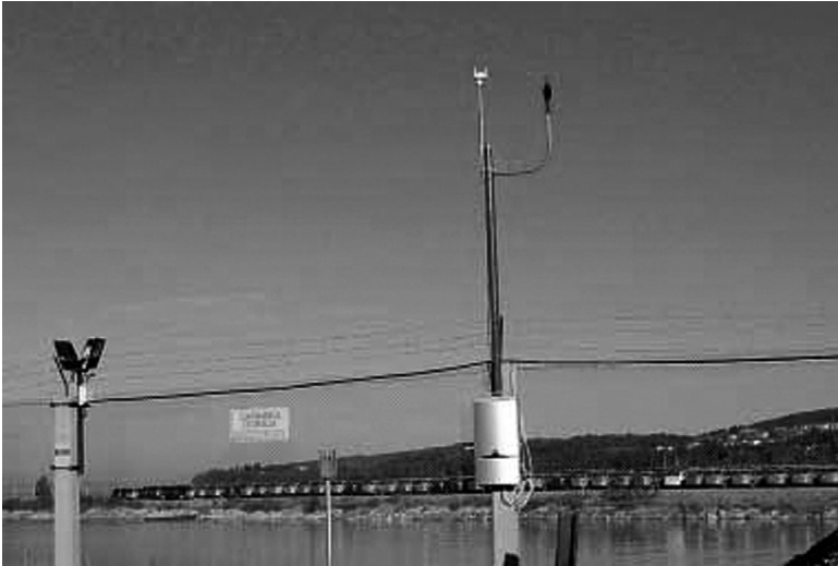
Figure 9: Equipment for continuous measurement of noise in the Port of Koper
