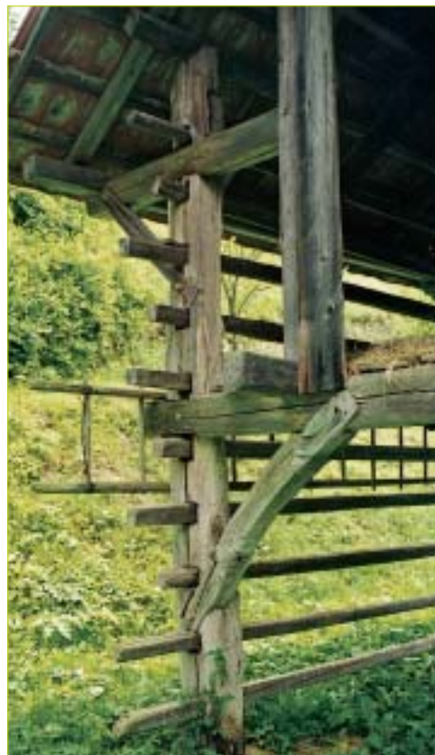
Detajl roke na kozolcu. Detail of the arm on the hayrack.
